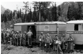
Mobile exchange on a train serves troops guarding 500 miles of Alaskan railroad.
